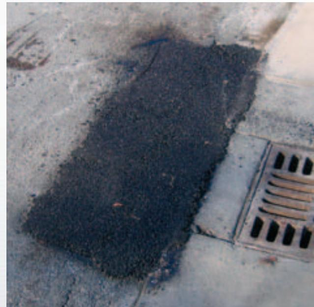
*With increased patch quality, Irondequoit saves 10 man hours some weeks producing new patches like this instead of performing repetitive repairs.*
