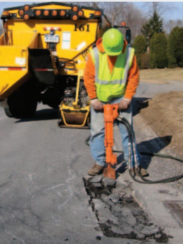
*A hydraulically driven pavement breaker located on the back squares off the pothole area.*
